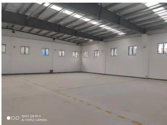
飞灰固化块暂存间地面防渗层
